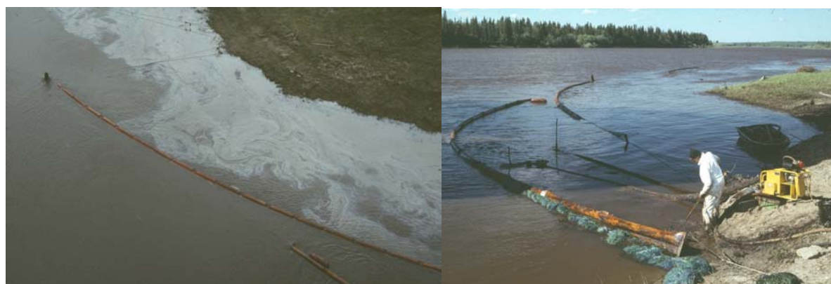
Figure 2 High-angle cascading diversion boom configuration in a fast current, Kolva River, Russia 1995. View from above (left) and at the river bank recovery location (right).
